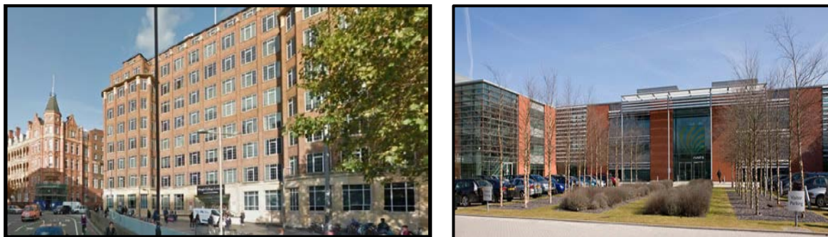
Figure 1 The two case study buildings: Case study 'K' (left) and case study 'N' (right)
