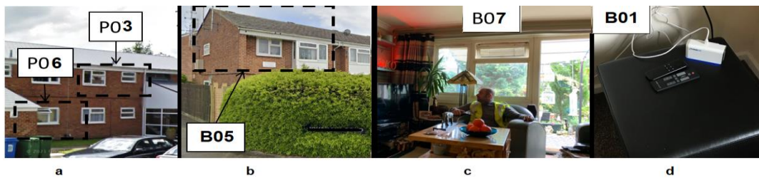
Figure 1. Examples of flats façades (a and b), living room space and Airthinx device (c and d)
