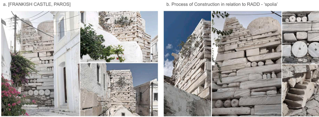
Fig. 1. Frankish Castle in Paros, Greece [29]. a. [FRANKISH CASTLE, PAROS] Constructed in 1260 during the Venetian occupation, the Frankish Castle was built atop the remnants of a 6th-century BC temple, utilising spolia—reclaimed stones from dismantled sanctuaries and ancient structures. Its construction demonstrates an adaptive reuse of available materials, driven not by stylistic preference but by the need to build using what was immediately at hand. The dry stone technique, which involves wedging stones together without mortar, further emphasises the response to material limitations and site-specific constraints. This technique was both practical as it accommodates irregular stone shapes, and reversible, allowing for potential future disassembly or repair. In summary, the Frankish Castle embodies a similar methodology to RADD where it was shaped by the availability of salvaged materials, the constraints of the site, and the novel method of reuse, resulting in a design that is contextually responsive, materially efficient, and historically layered. b. Process of Construction in relation to Resource Availability Driven Design (RADD): Surveying Existing Ruins + Material Stock - Selective Deconstruction - Sorting + Adapting Components - Dry Stone Const. Technique - Design Outcomes as Byproduct of Material Logic. The Design Language, the eclectic visual language of the castle, an irregular patchwork of classical and regular stone elements, was a direct result of material-led design, as it is not a stylistic intention. This aligns with the RADD principle that form emerges from resource constraints and availability, not from predetermined design ideals.
