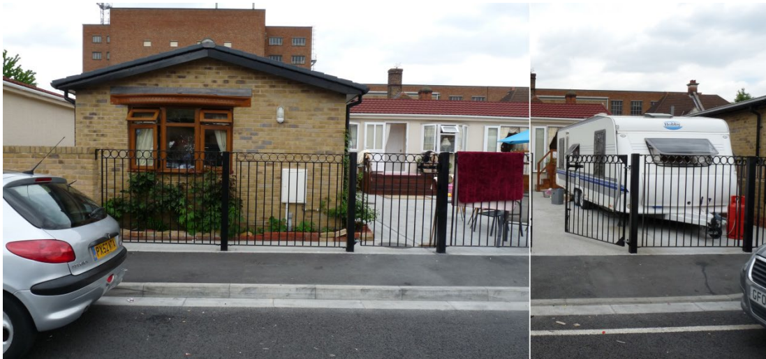
fig. 7.8 Image above, brick fixed structure as dayroom on left with chalet in background, and mobile caravan on right (2010)
