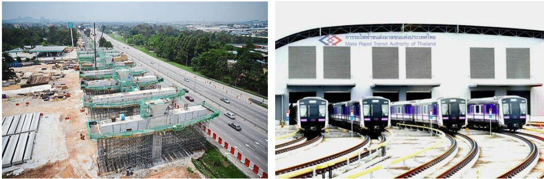
Figure 6.21 Overview of the construction works of (ICJV Project-2C).
