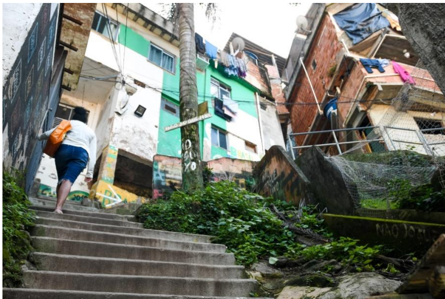
Figure 5: Steep staircases in Favela Santa Marta.
