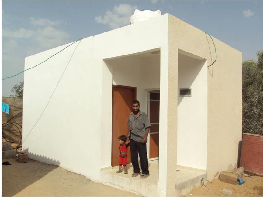
Figure 4.13: The project offered low-cost housing solutions for poor communities. Even the project's budget was limited, some units rendered and painted taking into consideration the future horizontal extension (rough render for external wall and smooth render for interior wall). Source: Salem Al Qudwa, 2011.
