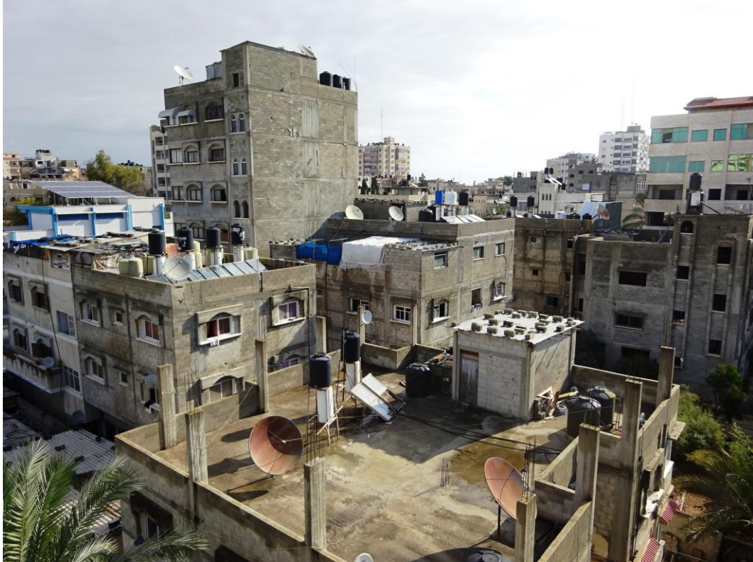
Figure 6.14: The picture conveys the over crowdedness of Gaza's urban landscape, as well as the incremental nature of erecting buildings. Source: Salem Al Qudwa, 2016.
