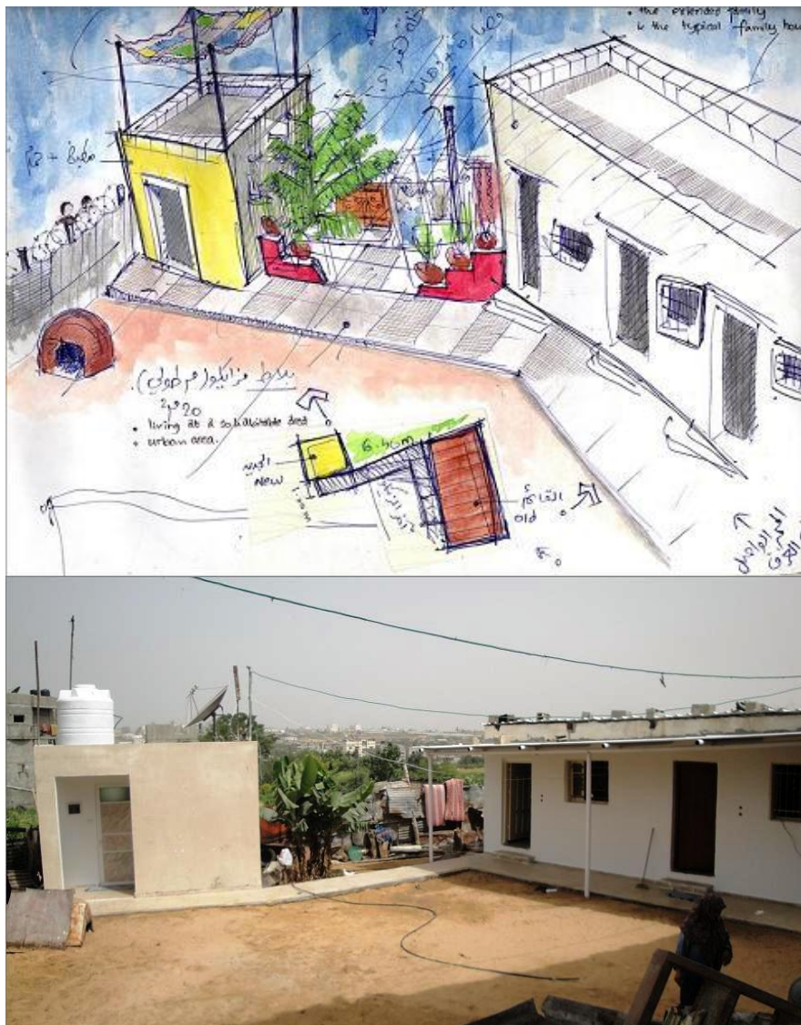
Figure 4.10: Sketch notebook and concrete were the media of communication at site. Source: Salem Al Qudwa, 2010.
