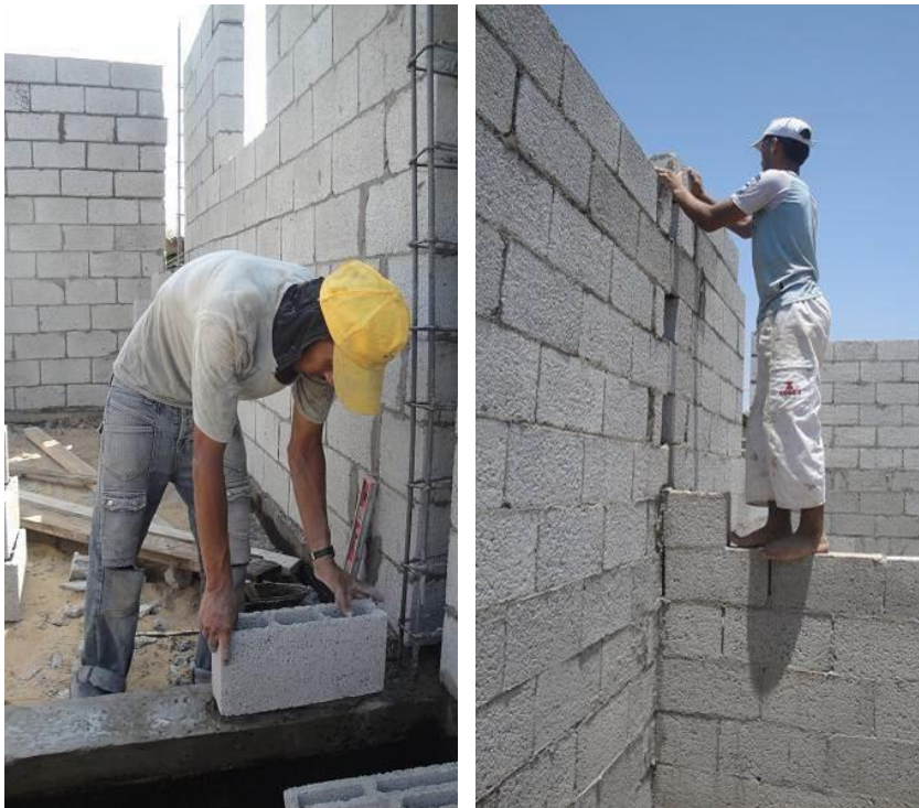
Figure 1.1: An example of a construction site in the Gaza Strip; and without being equipped with hard hats or lifelines, semi-skilled bricklayers peer down while putting another row of cement blocks. Source: Salem Al Qudwa, 2010.
