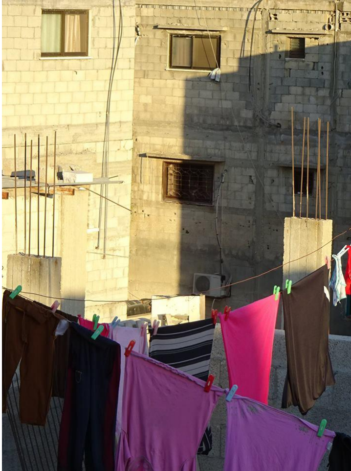
Figure 6.10: Some homeowners often do not complete the construction of the upper floor, as doing so prevents the reclassification of the building from ‘work in process’ to ‘completed building’. Often some of the support columns are used as planters or to hold laundry lines. Source: Salem Al Qudwa, 2016.
