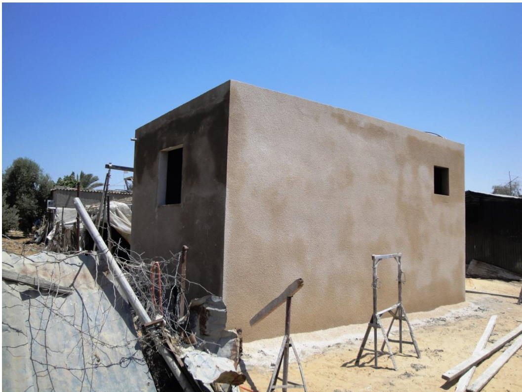
Figure 6.15: A simple breeze block structure that expresses the power and fragility of the architecture of the everyday in Gaza, while meeting local needs and budgets. Source: Salem Al Qudwa, 2010.
