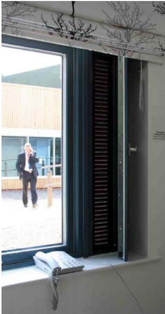
Figure 10 – Louvered window proving safe ventilation.
