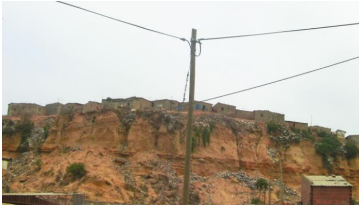
Fig 3.10 - Bairro Samba, built on a risk area where various landslides have already occurred, destroying many houses. Photo by Célia Macedo, 2011.
