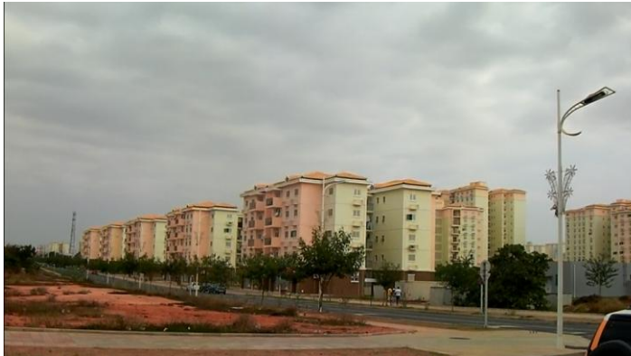
Fig. 3.12 - New city built on the outskirts of Luanda – Kilamba Kiaxe under construction. Photo by Célia Macedo, 2011.
