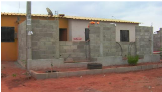
Fig. 7.3 - Example of house in Zango 4. typical occupant intervention to increase living area. Ongoing construction of an extension to increase area of the house. Photo by Célia Macedo, 2013
