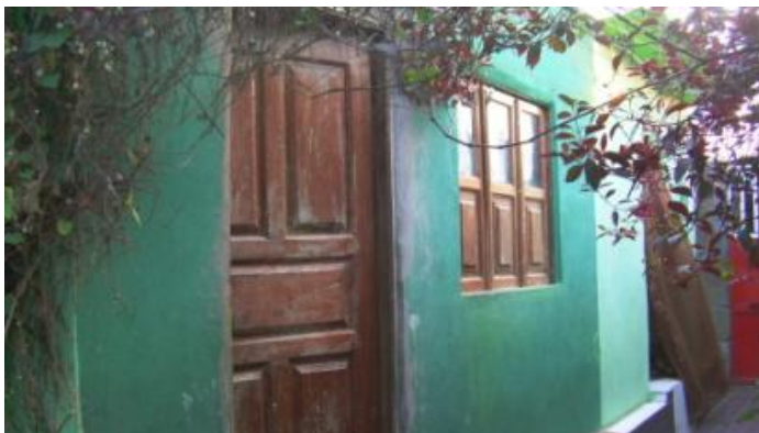
Fig. 8.2 - CHIC-3:M, Type 1a. External view, main entrance. Use of colour and plants to adorn the façade. Case Area One. Photo by Célia Macedo, 2011
