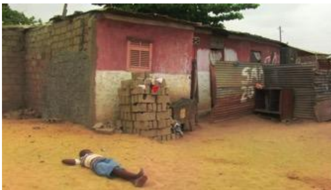
Fig. 2.19 - Concrete block house - Bairro Cazenga, Luanda. Photo by Célia Macedo, 2011
