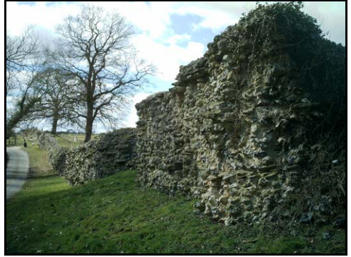
View of the wall from Church Lane, just past the church
