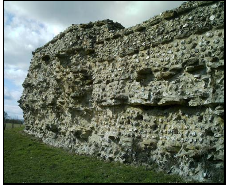
View of the wall from the south side
