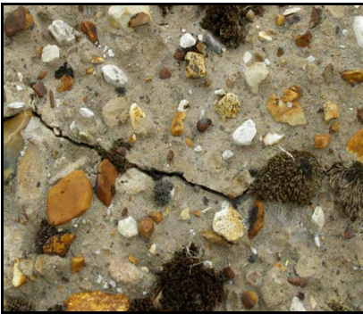
Example of mortar infilling on the wall
