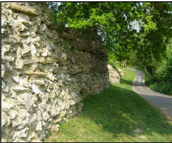
View of the wall from Church Lane
