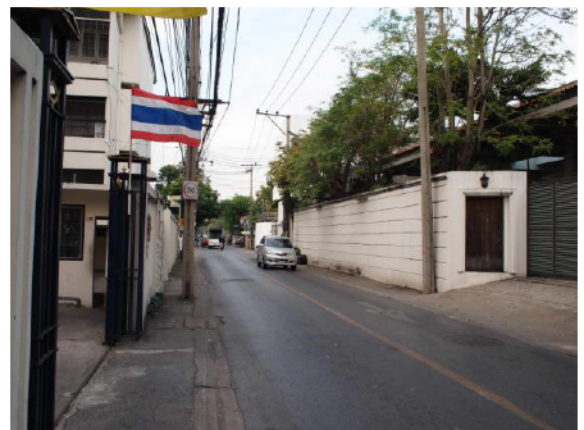
Solid fences built to clearly separate public and private spaces
