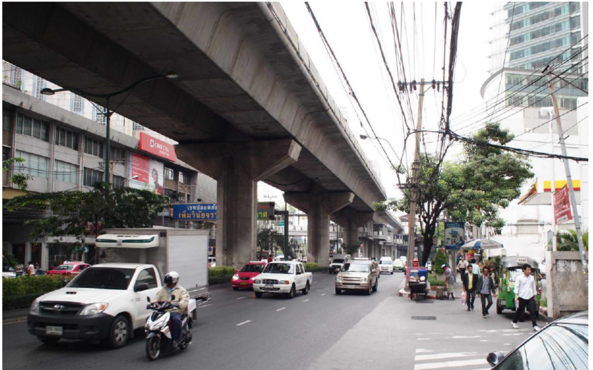
Figure 8.4 The Construction of the Elevated Railway Above Sukhumvit Road, 2012 Source: Author, 2012
