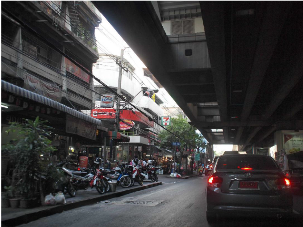
Figure 6.12 The Construction of the Elevated Railway above Sukhumvit Road, 2010 Source: Author, 2010
