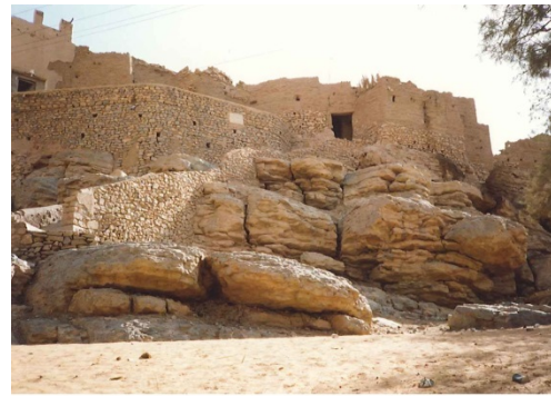
Figure 3. Rocky site on which the Ksar of Taghit was built. Bottom part of walls built with stones joined with earth-based mortar.
