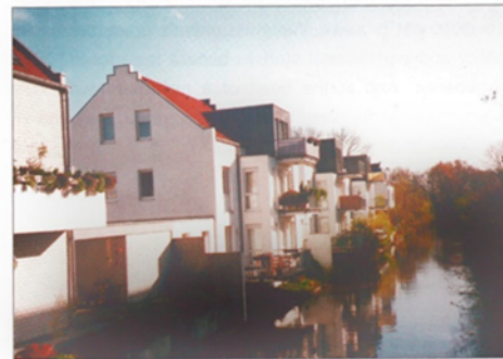
German design and construction skills in evidence in Norderm
