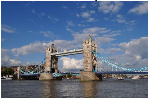
Figure 1. 5: Tower Bridge Source: Ren, 2014
