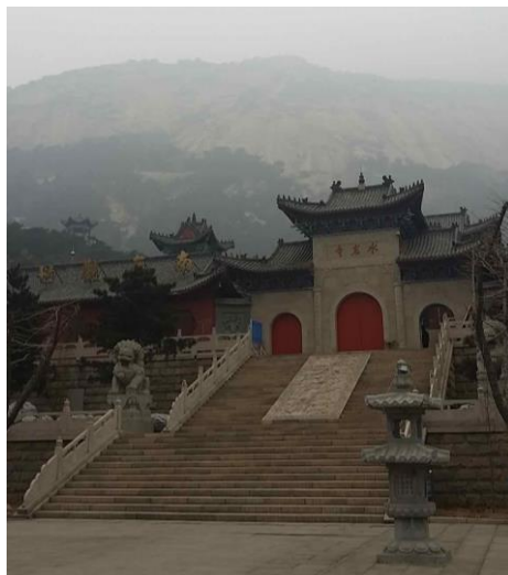
Figure 5. 27: Gate of WRT, 2015
