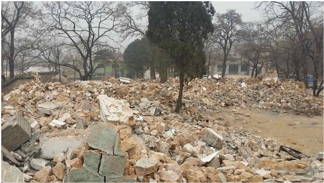
Figure 5. 42: The army building's ruins in front of WRT, 2015
