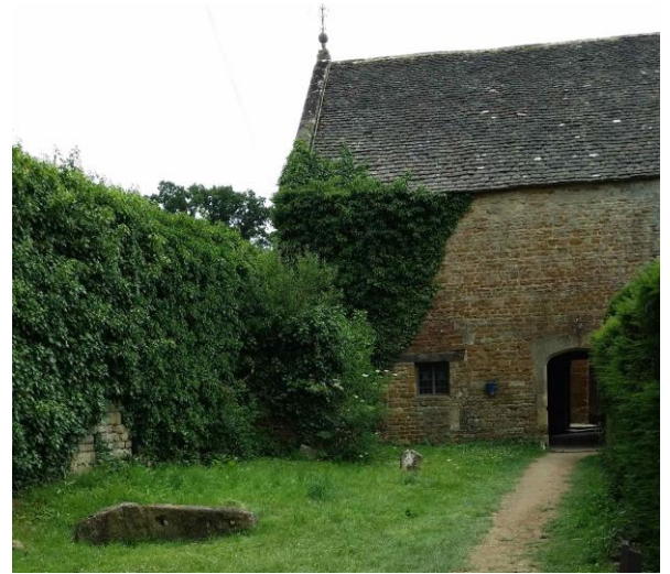
Figure 5. 6: Historic building in Chastleton Garden, 2013
