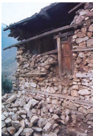
Figure 4.4 Traditional building with wooden tie beams
