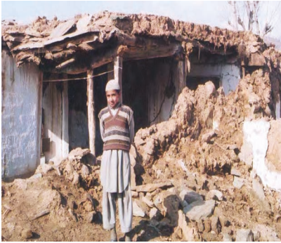
Figure 4.1 Heavy roof construction held up by wooden posts
