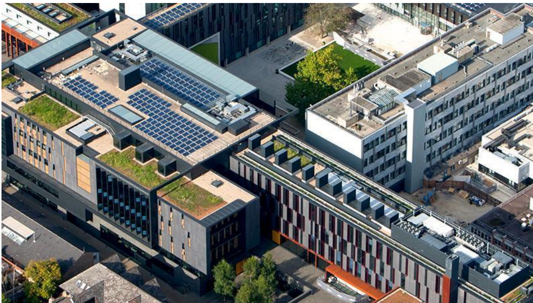
Figure 9.6: SunPower Modules Installed on an Oxford Brookes University Building [source: (Oxford Brookes University, 2020)]
