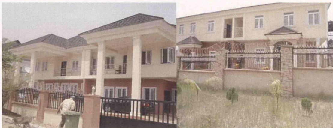
Figure 4.12: Fully completed EPS houses showing the front and rear view from left to right (Location: CITEC Abuja, photographed by the author).
