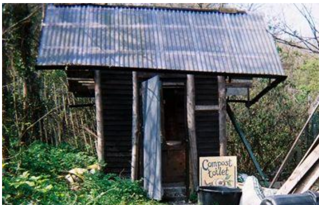
Figure 7.24: The Compost Toilet
