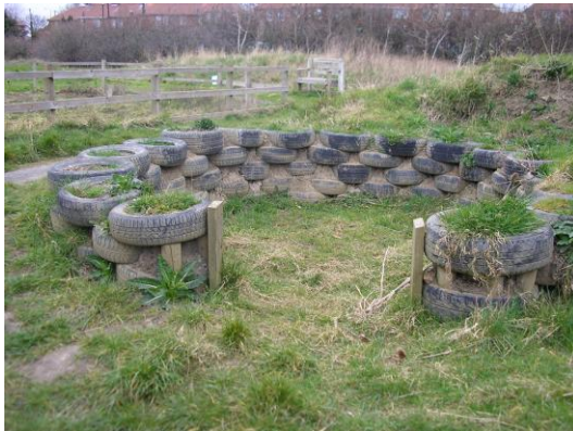
Figure 7.28: Reuse of old tyres to create a play area
