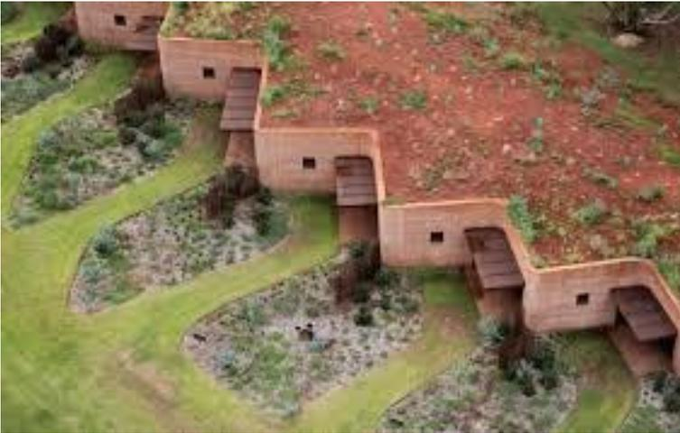
A technique that can be used to construct foundations as well as walls and other materials by either packing earth into a wall framework where different layers are added at different stages. This method dates back to 5000 BCE
