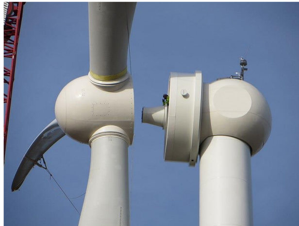
Figure 3: A gearless wind turbine rotor of HWAT [14]
