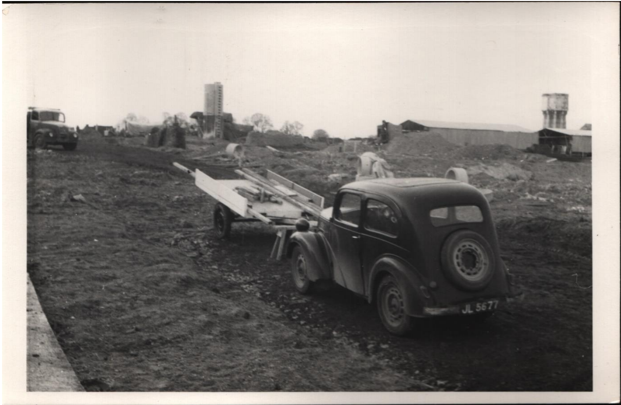
Image 25: Building Work for Westminster College Oxford.
