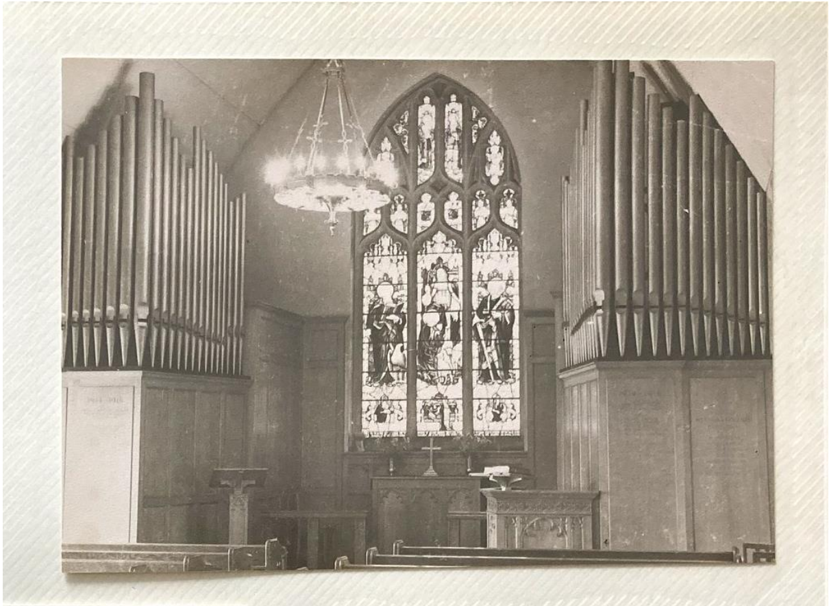
Image 20: Restored Chapel, c1950.
