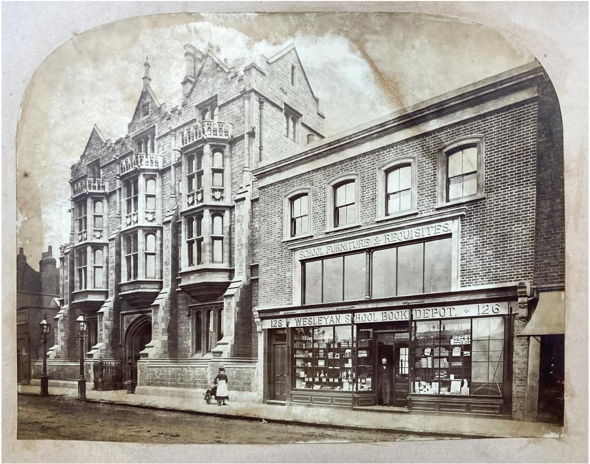
Image 3: Exterior of Westminster College, facing onto Horseferry Road.
