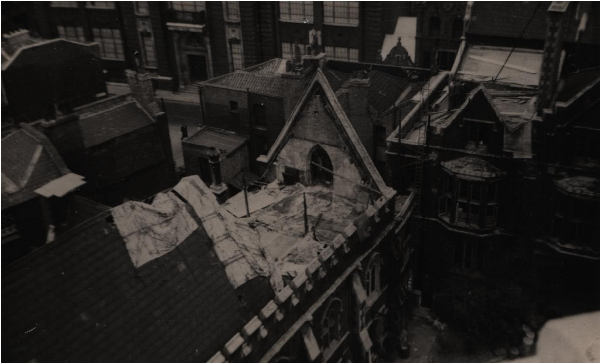
Image 15: Bomb damage to the Chapel, 1944.
