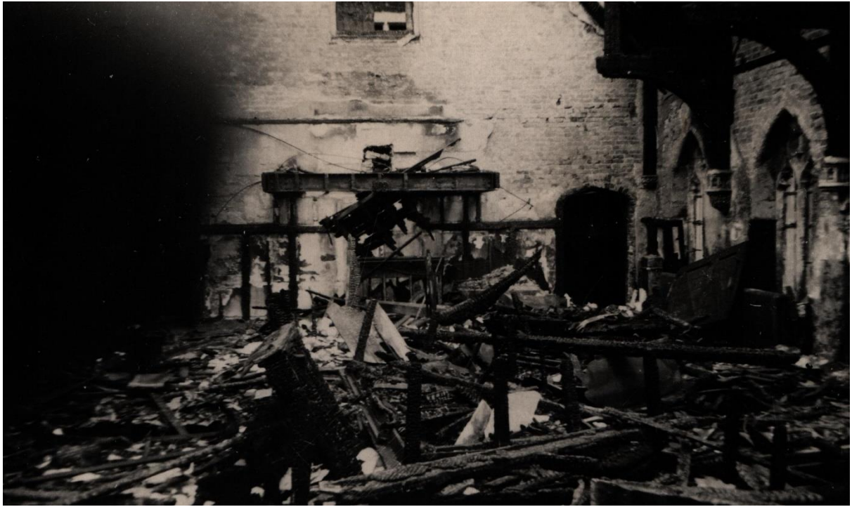
Image 16: Bomb damage to the Dining Hall, 1944.
