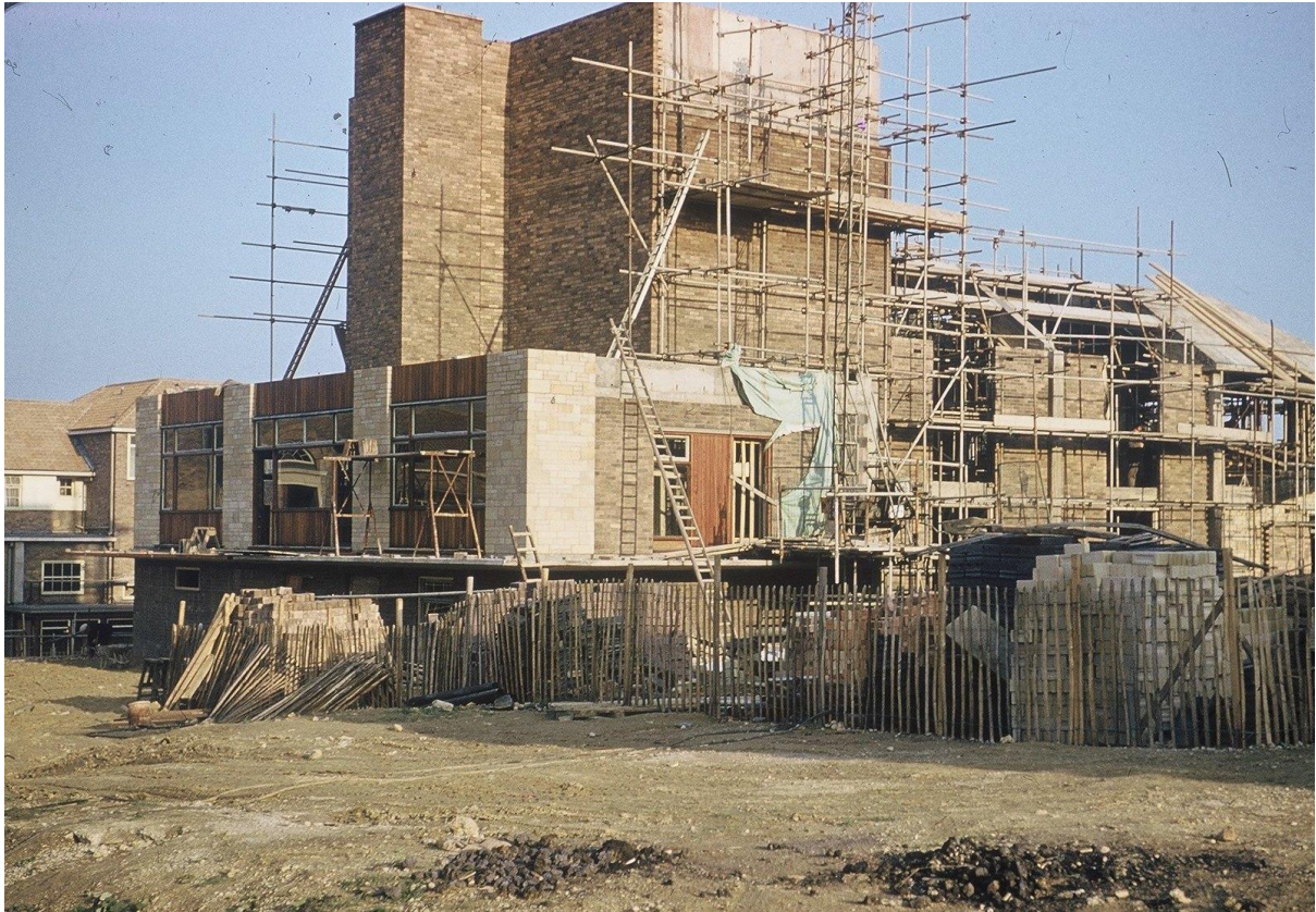
Image 28: Building the main Lecture Theatre.
