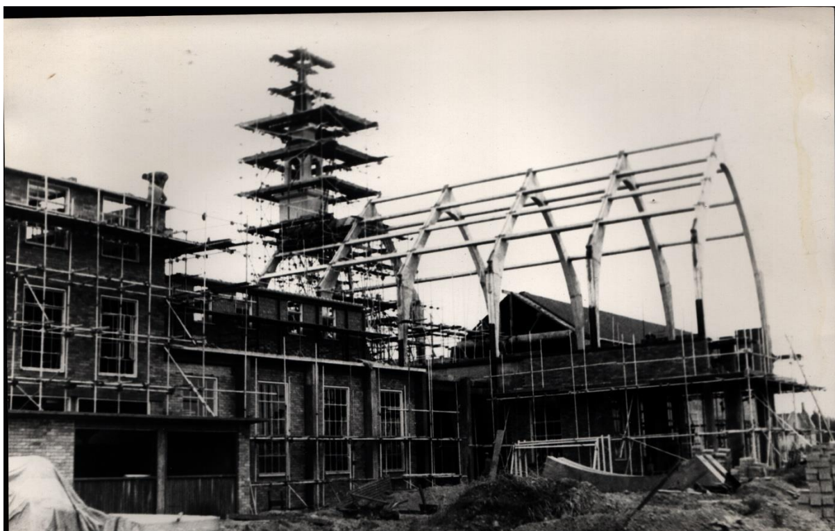
Image 26: Erection of the College Chapel.
