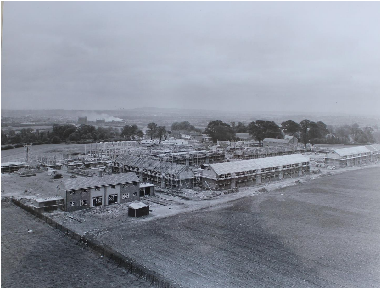
Image 27: Building Student Accommodation.
