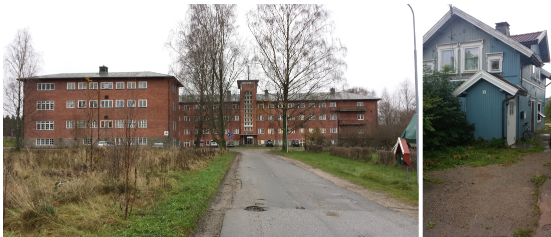
Fig. 1. Centralised centre Elvestad (left) and decentralised accommodation (right). (Photos by Thorshaug)
