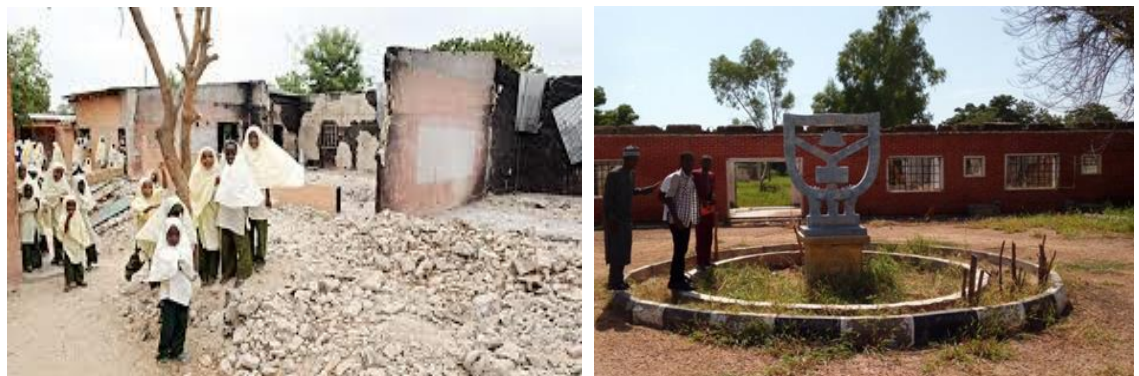
Figure 7.3: Post-conflict condition of schools in Buni Yadi
