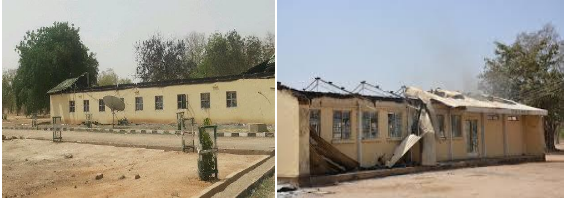
Figure 7.8a: Destroyed local government offices after the conflict in Buni Yadi
