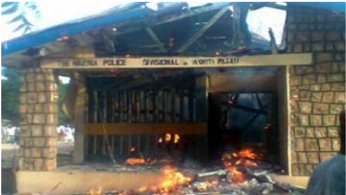
Figure 7.8b: Vandalised police station in Buni Yadi
