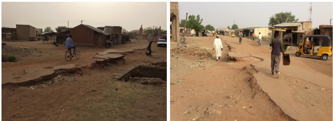
Figure 7.5b: Damaged road in Buni Yadi after conflict.
