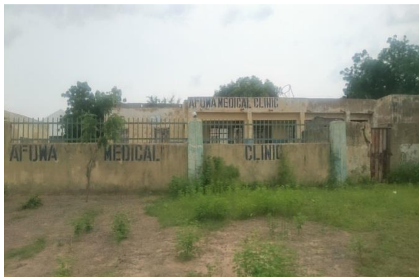
Figure 7.4: Post-conflict condition of hospitals in Buni Yadi
