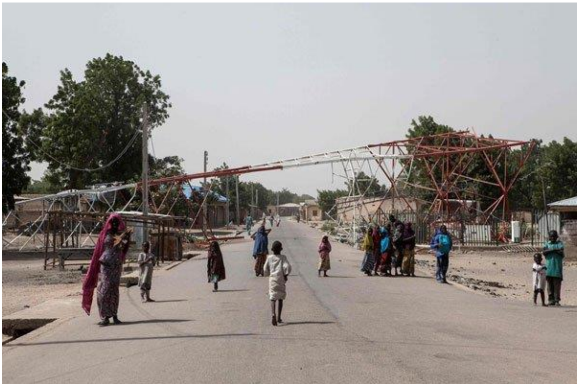
Figure 7.7b: Vandalised telecommunication infrastructure after the conflict in Bunia Yadi
