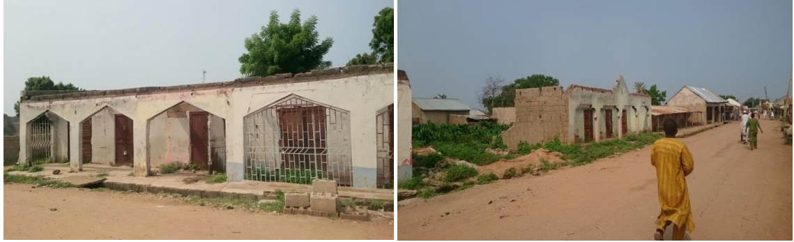
Figure 7.2: Post-conflict condition of shops and stores in Buni Yadi
