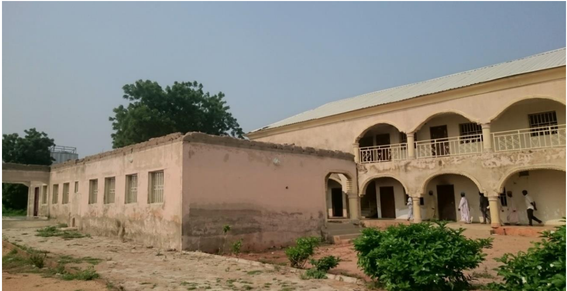
Figure 7.8c: The destroyed palace of the Emir of Buni Yadi after conflict.
