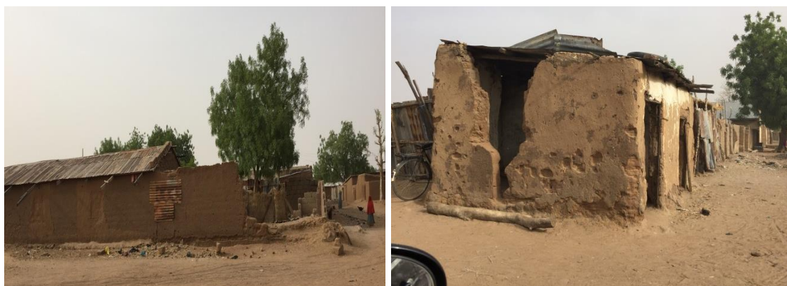
Figure 7.1b: Post-conflict condition of mud-block houses in Buni Yadi
