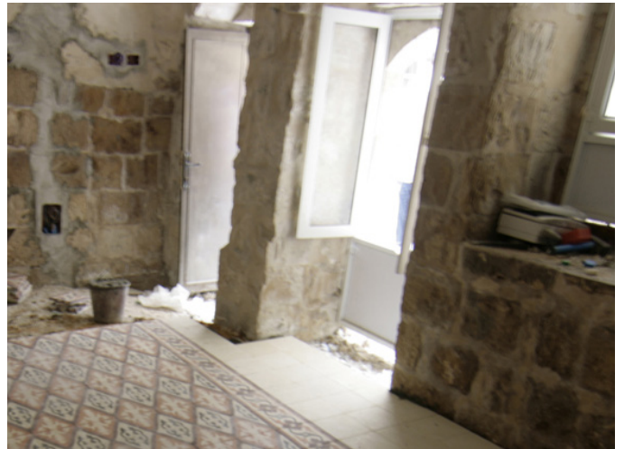
Rehabilitation of the Bait al Karama women centre
