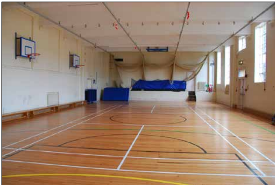
Fig. 35: Interior of Existing Sports Hall (September, 2013)
