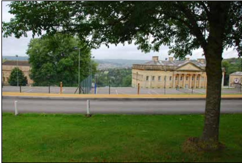
Fig. 44: View North over Mansion from Sports Pitches (September, 2013)
