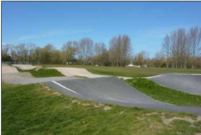
Fig. 80b: 'After': View North from Eastern Boundary of BMX Track (April 2013)
