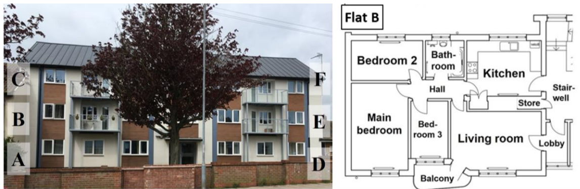
Figure 1 Case study flats (post-retrofit): east facade (left), representative floor plan (right).
