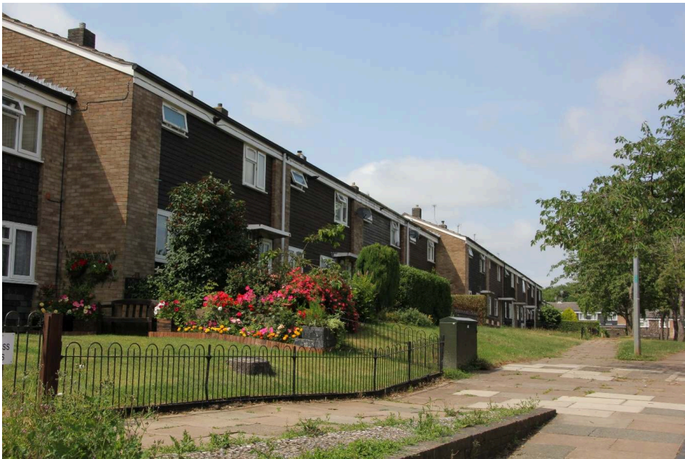
Figure 6: Mowlem system-built housing at Pin Green (Neighbourhood 6), built in approximately 1965. The area was laid out on the "Radburn" principle, with complete separation of vehicular and pedestrian circulation systems. This image shows the pedestrian-side.
