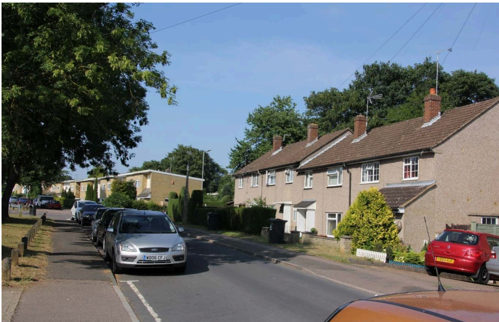
Figure 5: Foreground shows Wimpey 'no-fines' system-built P77-type housing in the Broadwater area of Stevenage (Neighbourhood 3), developed from 1953. Behind can be seen flat roofed housing of the Development Corporation's C23-type built shortly afterwards.
